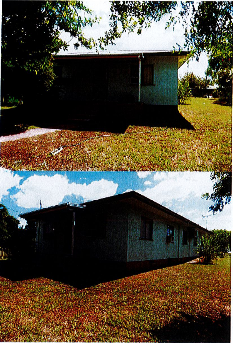
Front and side of house. Disabled ramp and access.
