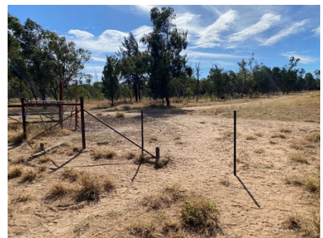
Botanical Reserve fence repaired
