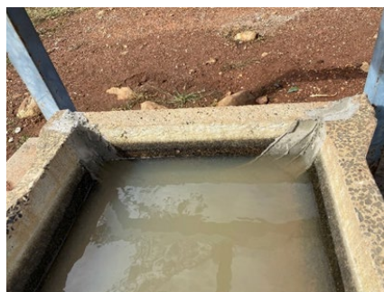
Trough repairs at Clara Creek Route
