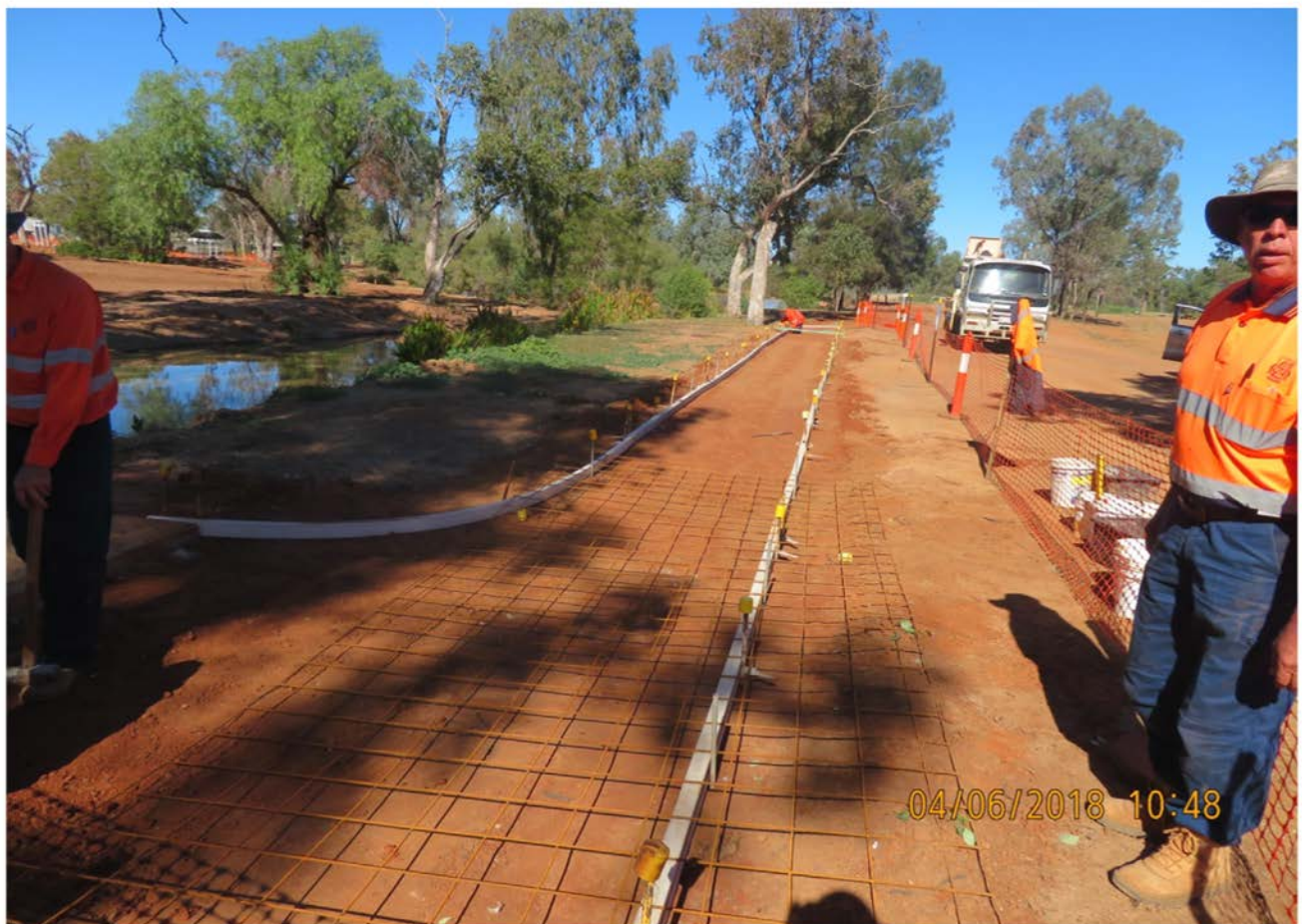
Installation of new footpath at Graham Andrew's Park.
