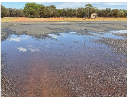
Ponding of water on the main runway Charleville Airport
