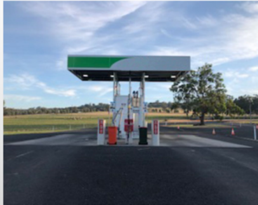
UNMANNED HYDROGEN REFUELLING STATION
