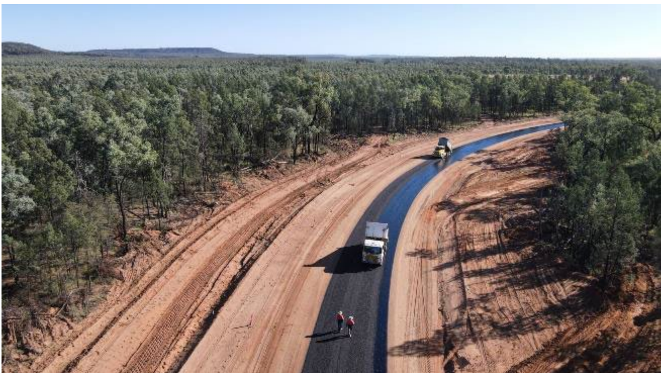
Sealing works on Mt Tabor Road (TIDS/R2R funded project)
