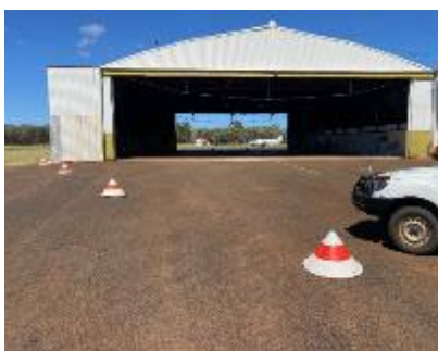
Roof repaired – damage caused in December 2023 wind storm
