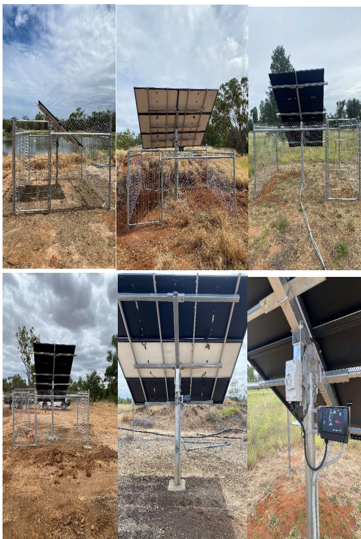
Capital Works completed
