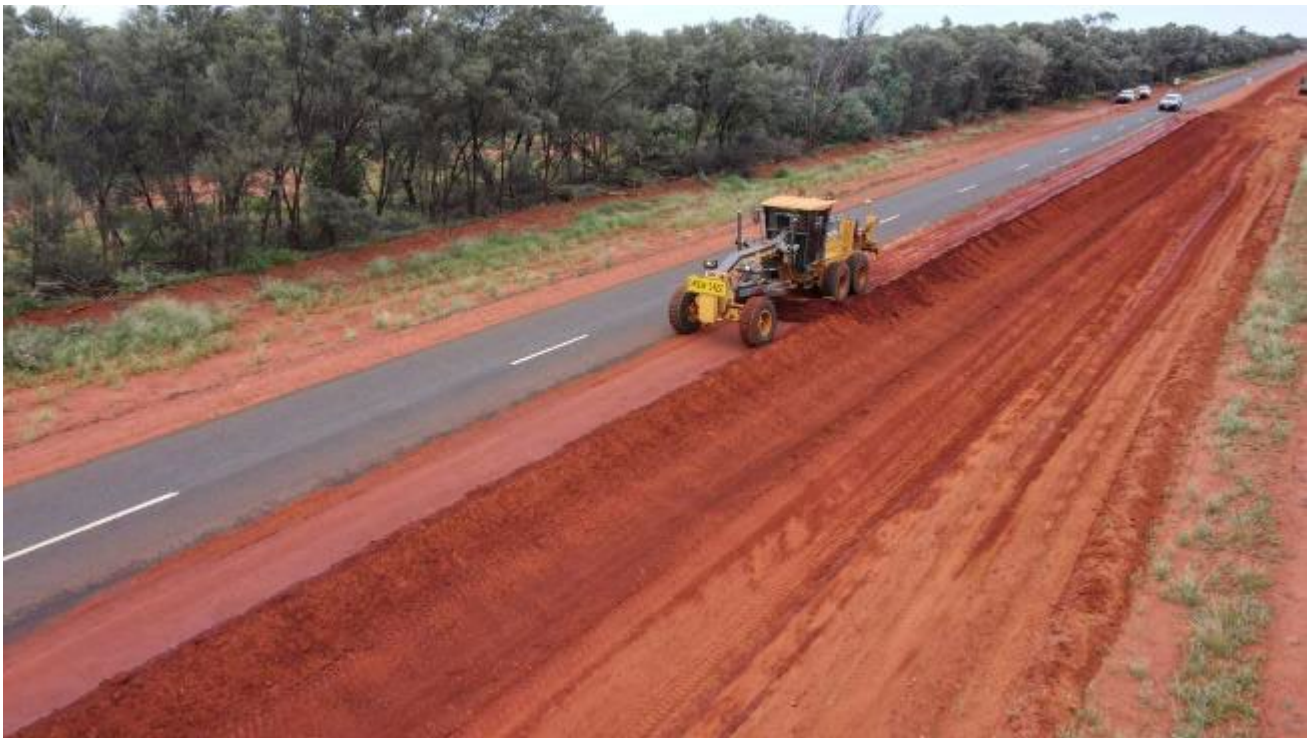
Shouldering works on the Mitchell Highway (Cunnamulla-Charleville)
