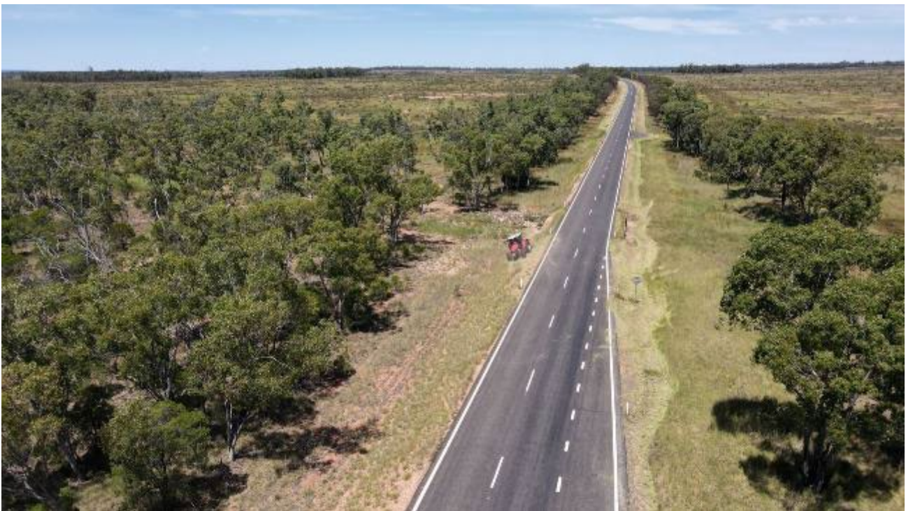
Slashing on the Landsborough Highway (Morven-Augathella)
