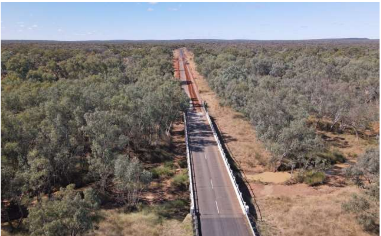
Stabilisation Works on the Diamantina Development Road (Charleville-Quilpie)
