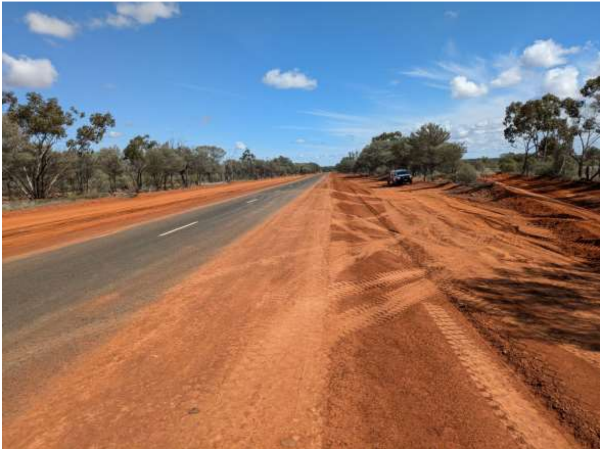
Shouldering works on 93A Diamantina Developmental Road (Charleville-Quilpie)
