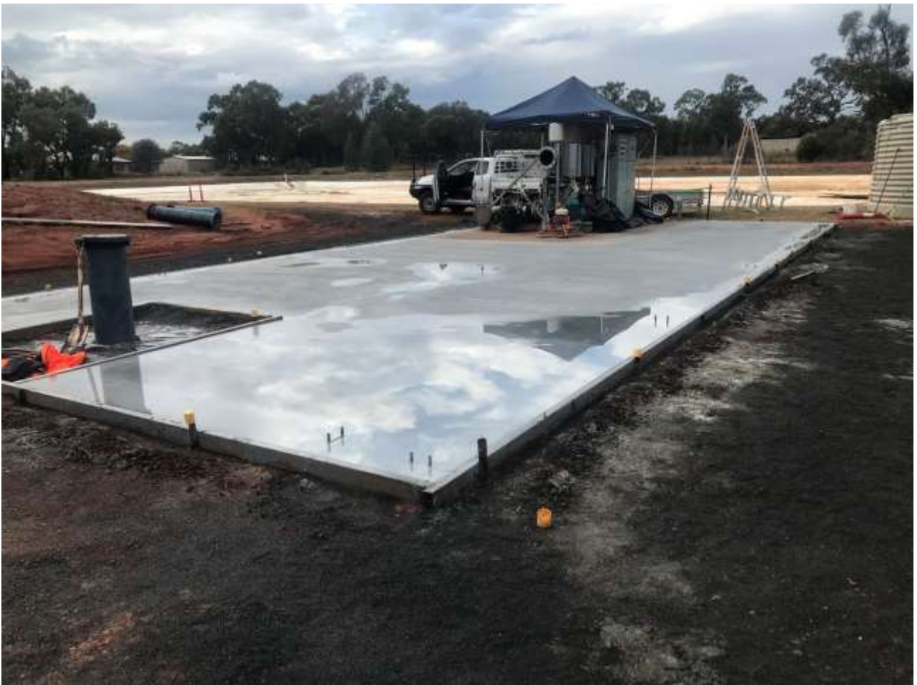
Concrete slab for new UV disinfection unit
