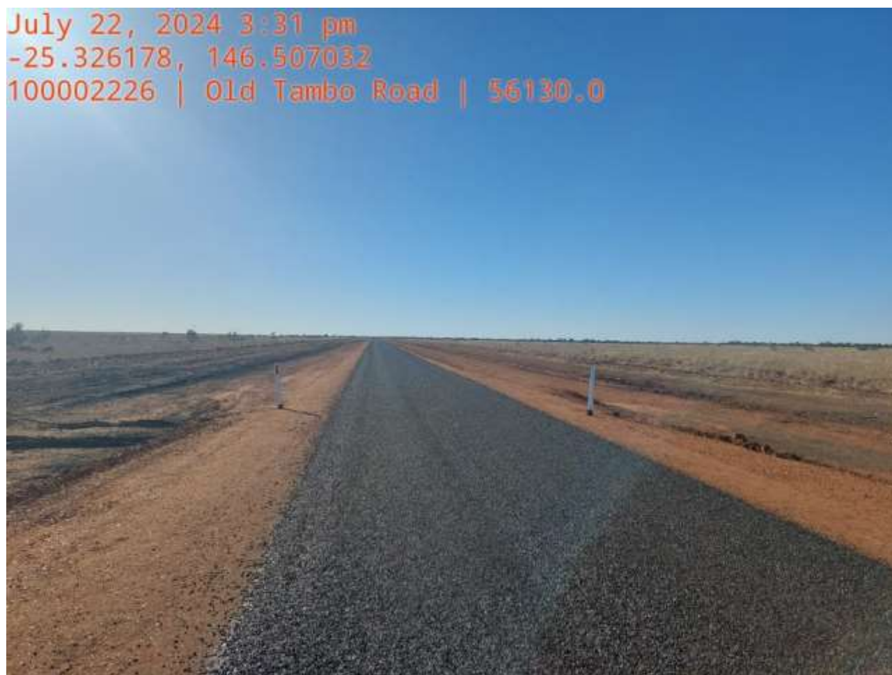
Completed sealing works on Old Tambo Road (Funded by LRCI Phase 4)
