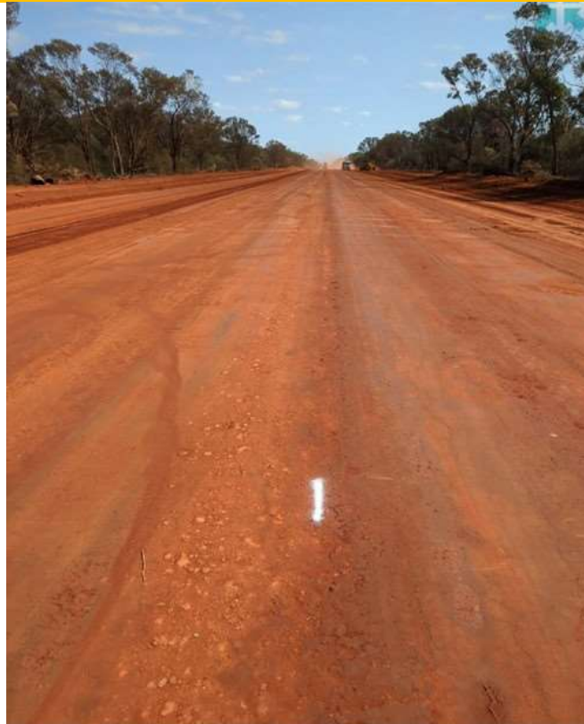
Adavale Road Re-Sheeting Project has Commenced funded by TIDS/R2R
