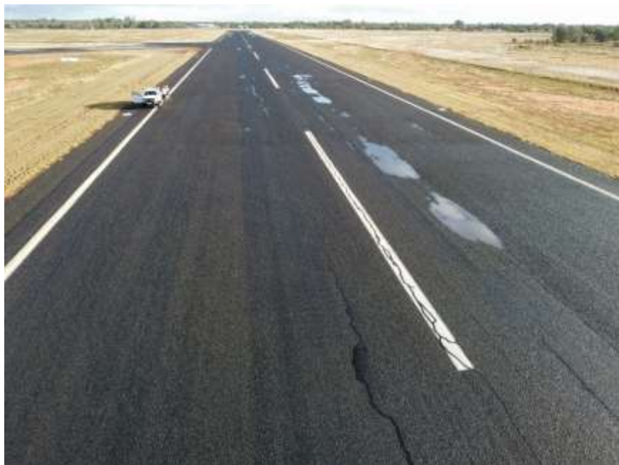
Drone image of runway 12/30 – sections of ponding water
