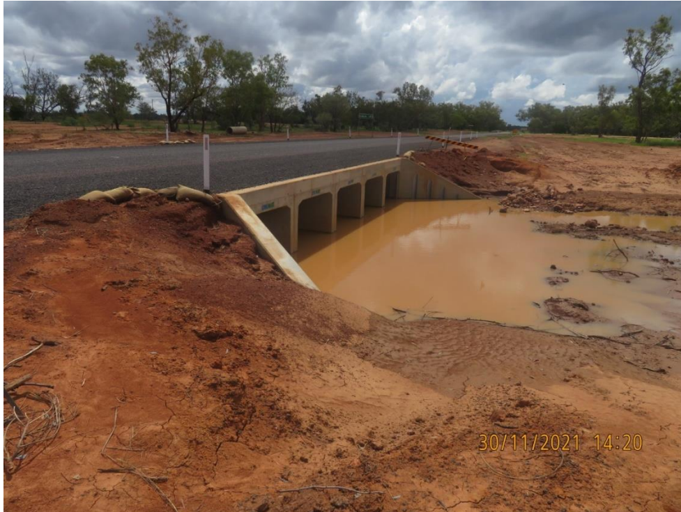
Cooladdi culvert replacement – Quilpie Road
