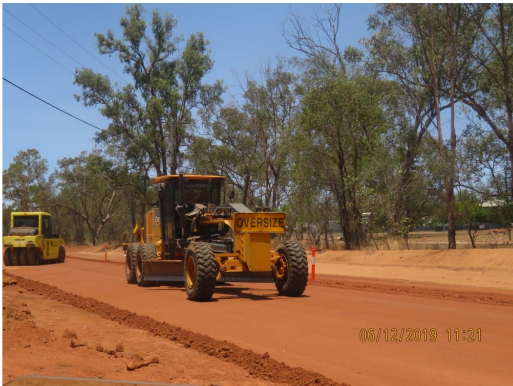
Carter St – preparation for sealing
