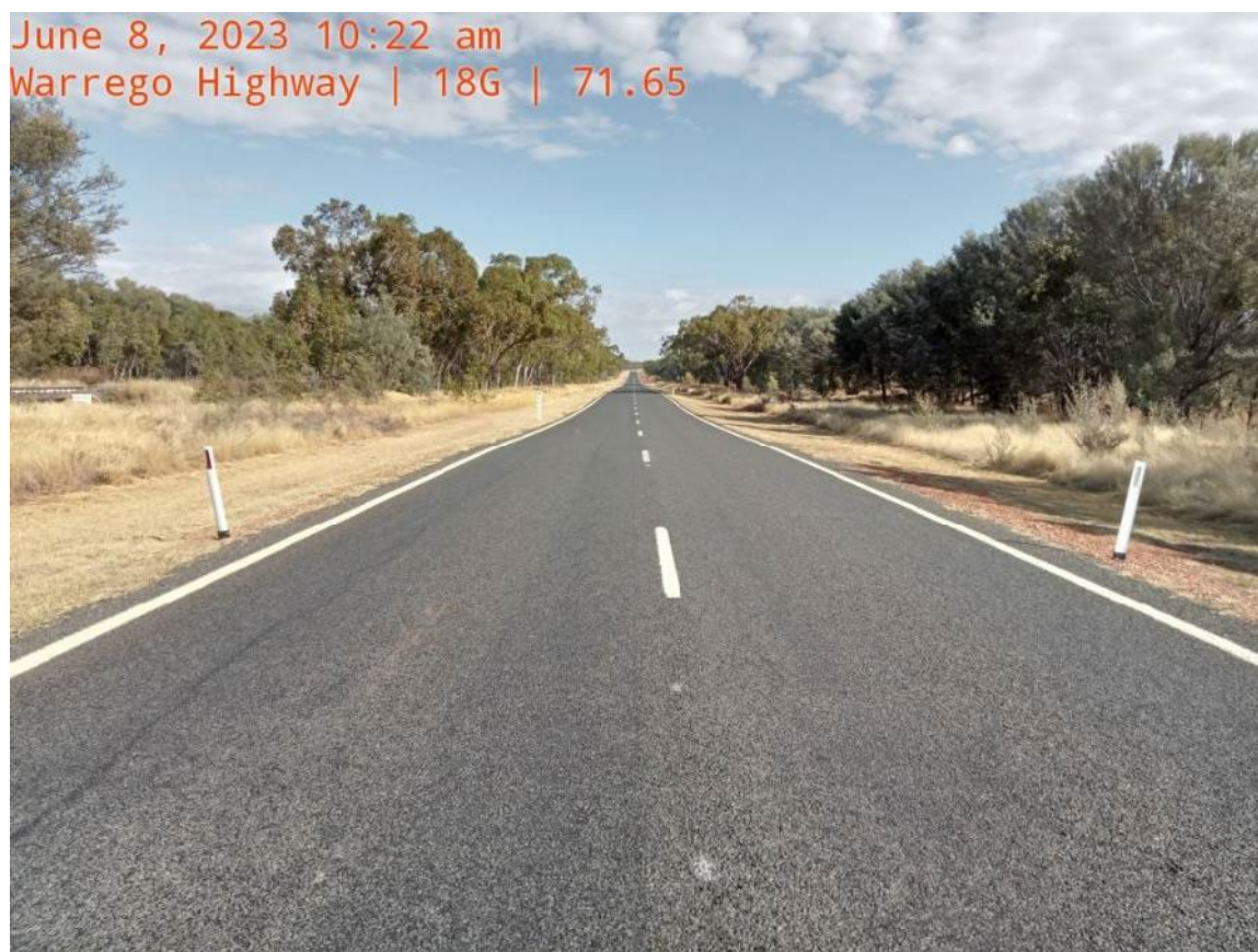
18G Warrego Highway (Morven – Charleville) Completed Slashing Works
