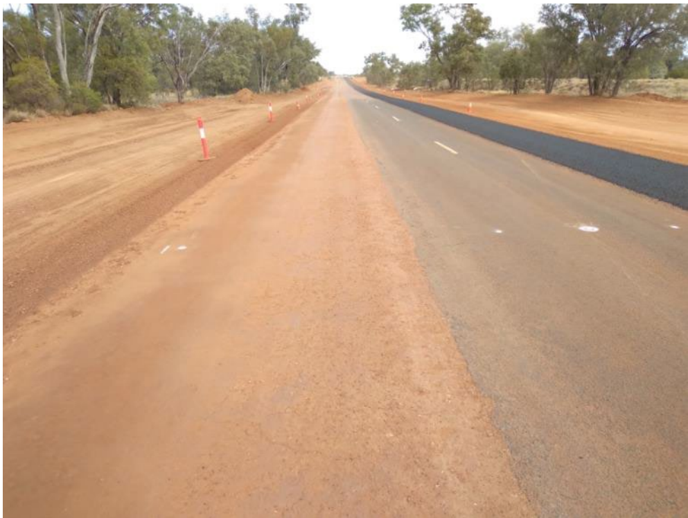
Mitchell Highway (Cunnamulla-Charleville) Upgrade Project
