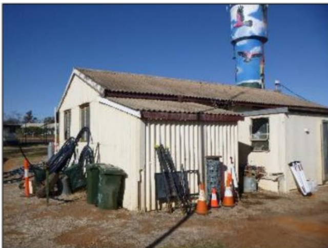
Unpainted damage, back corner of small side storage room.
