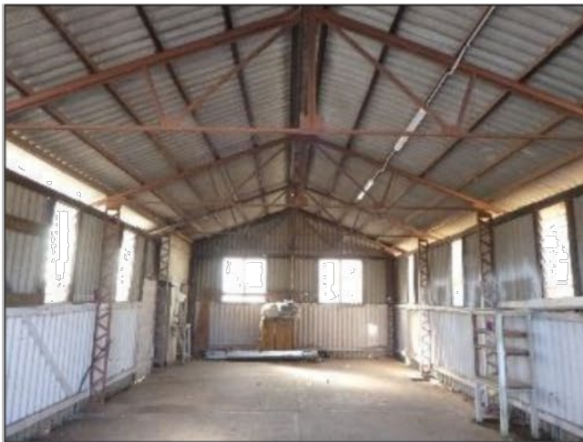
Internal roofing & walls.
