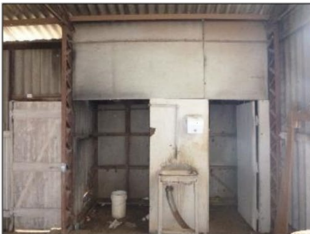
Inside, rear left corner, unpainted sheeting, toilet / shower.
