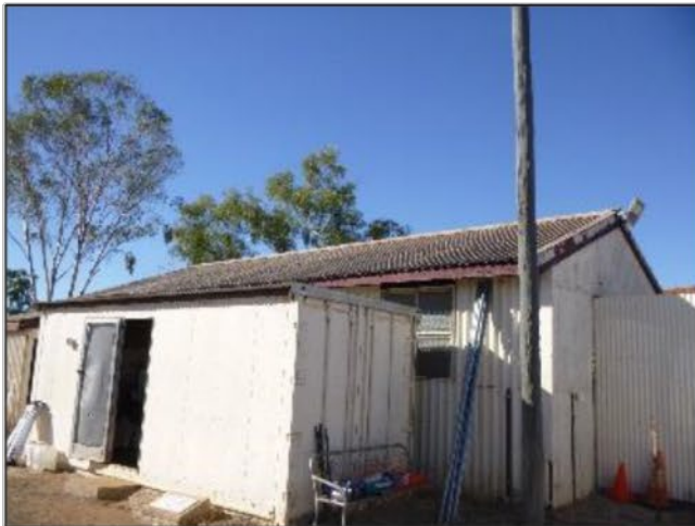
Unpainted roofing & top capping.
