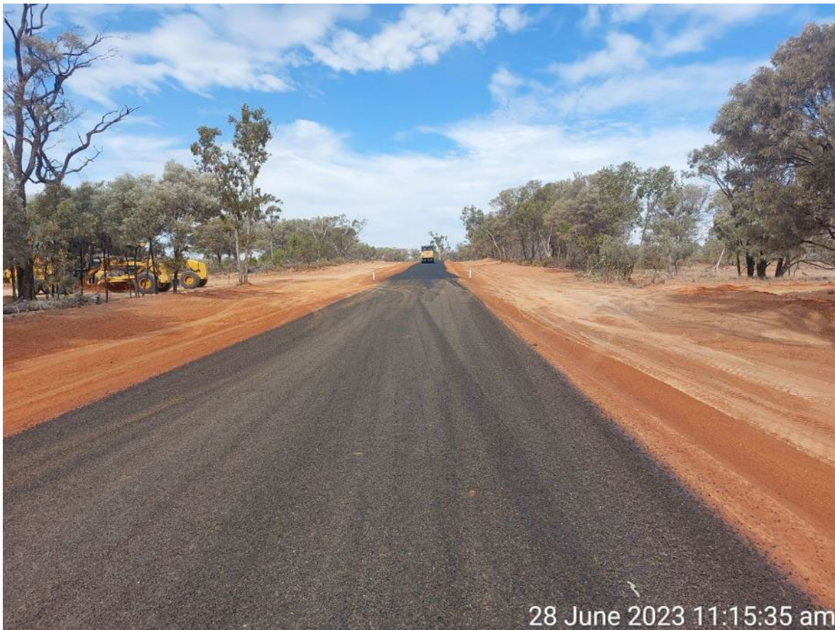
Langlo Mount Morris Road Sealing Works
