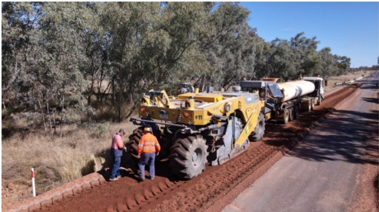
Stabilising Works being conducted on State & Federal Roads
