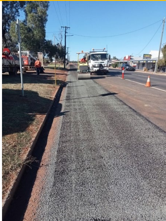
Morven Water Main Renewal Roadworks
