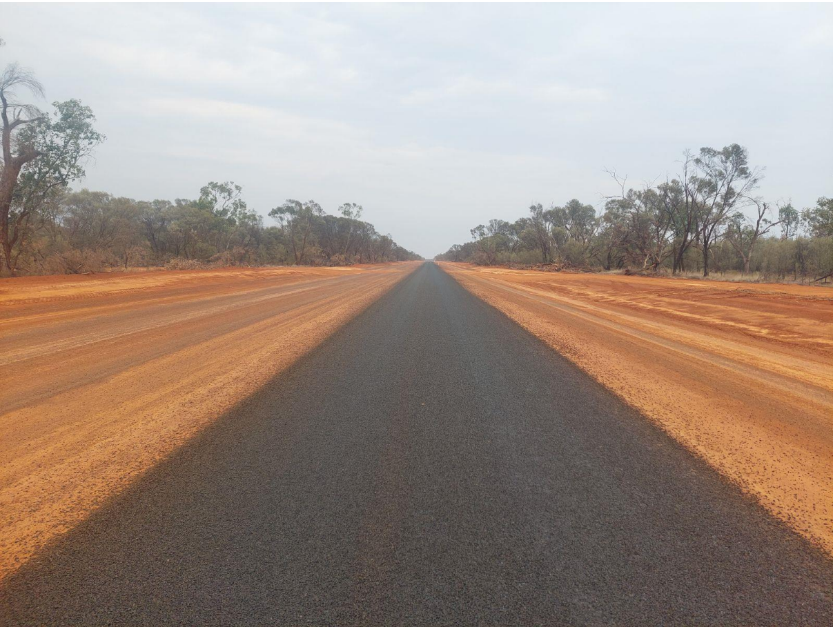
Adavale Road Sealing (TIDS/R2R Project)
